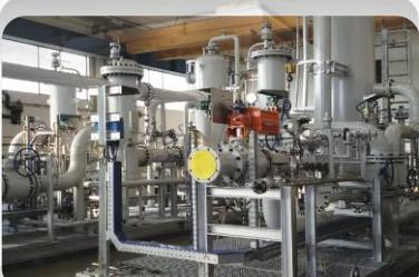
Pig launching and Receiving Traps - Gas pressure Reducing Station and Control Units - Skid Mounted Gas, Filtering Regulation, Metering
